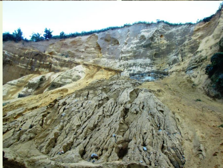
Banderdewa Mudslide Arunachal Pradesh 2013
