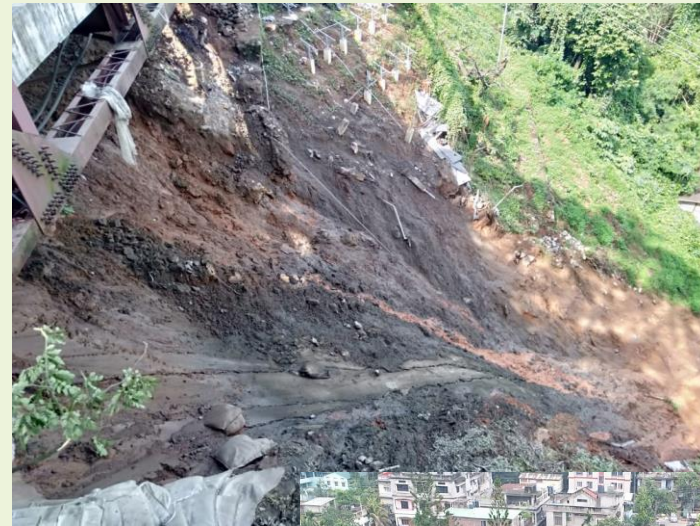
Landslide beneath Raj Bhawan Guwahati
